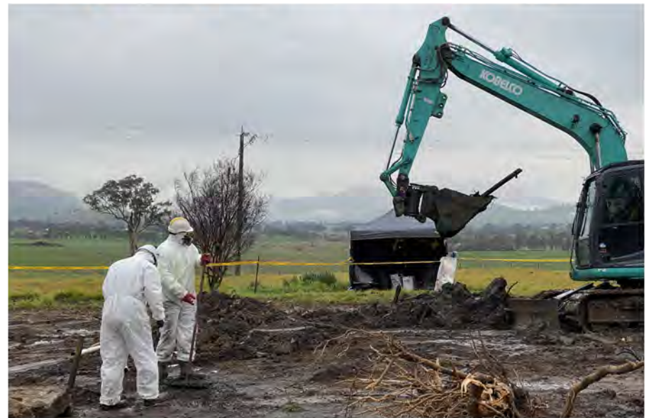
Grocon crews work to clear a dairy outside Cudgewa
